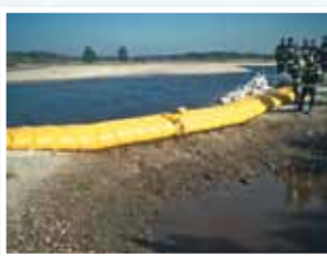
tightness of the interface between dams
