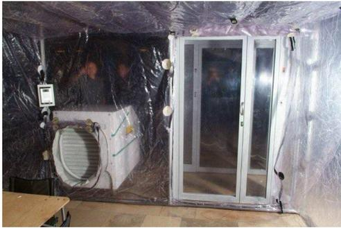
Inside of the isolation room – view to the sanitary lock and filter
